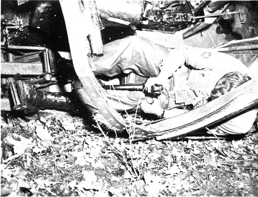
Figure 12. Posed photograph shows position of the copilot when the helicopter came to rest. Note the position of the copilot's head against the cockpit support member.
