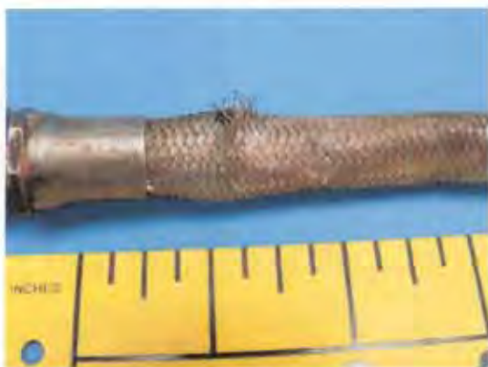
Ruptured flex line – CP11
