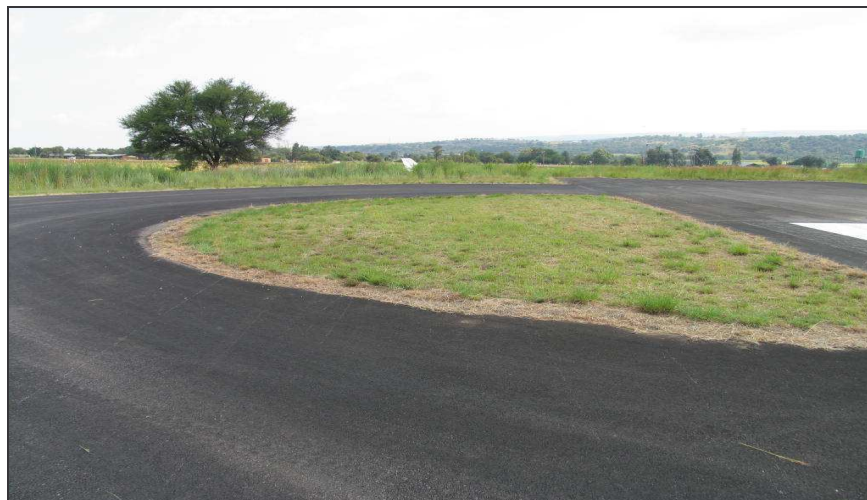
Figure 7. View of where the aircraft overran the end of the runway.
