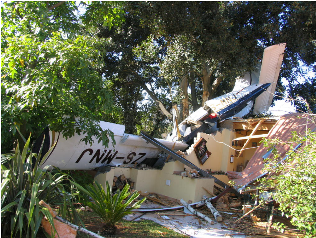
Figure 4. Another view of the damage to the entertainment area and the aircraft.
