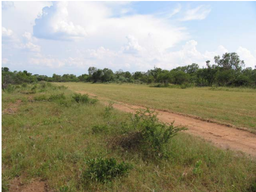
Figure 4. A view of the runway taken in the direction of the threshold of Runway 35.
