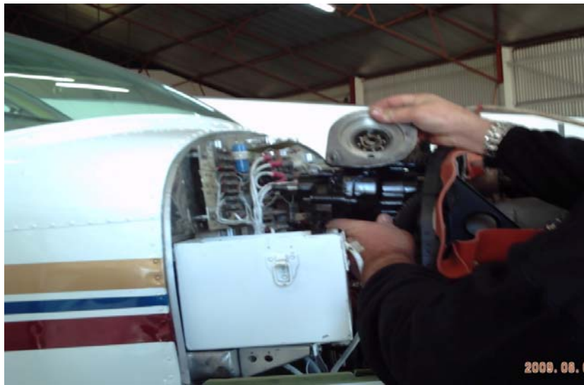
Picture 4 showing some of the challenges of installation.
