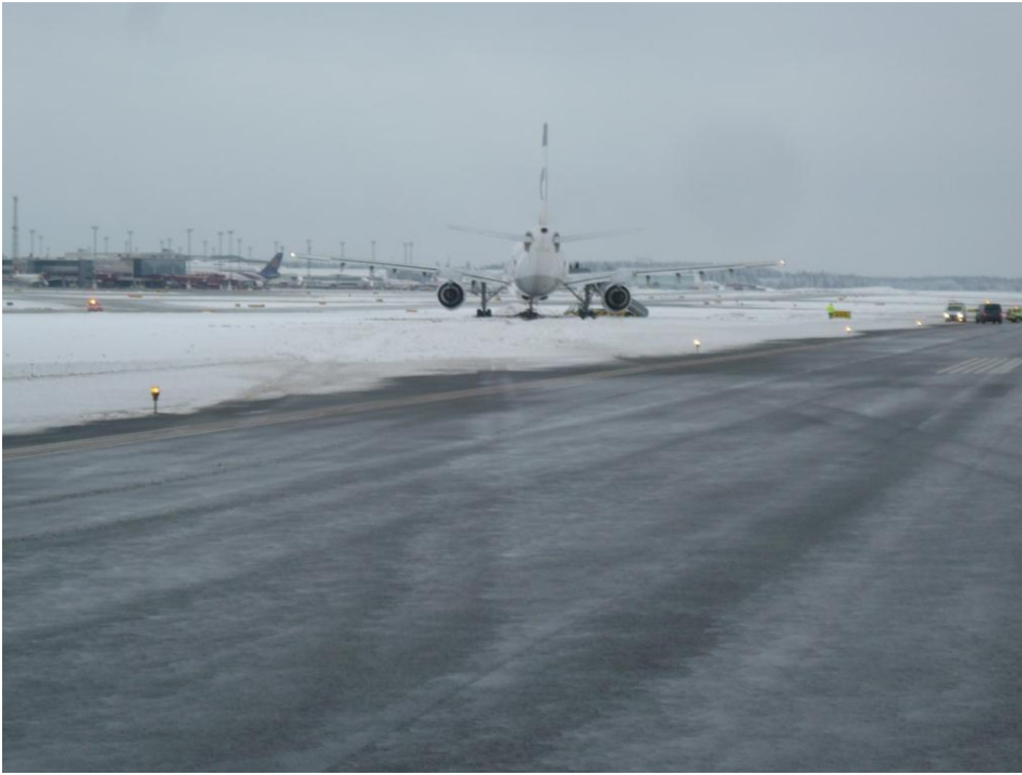
Fig. 50. (See also fig. 35b). Tracks on the contaminated runway surface. Photo: Swedavia.
