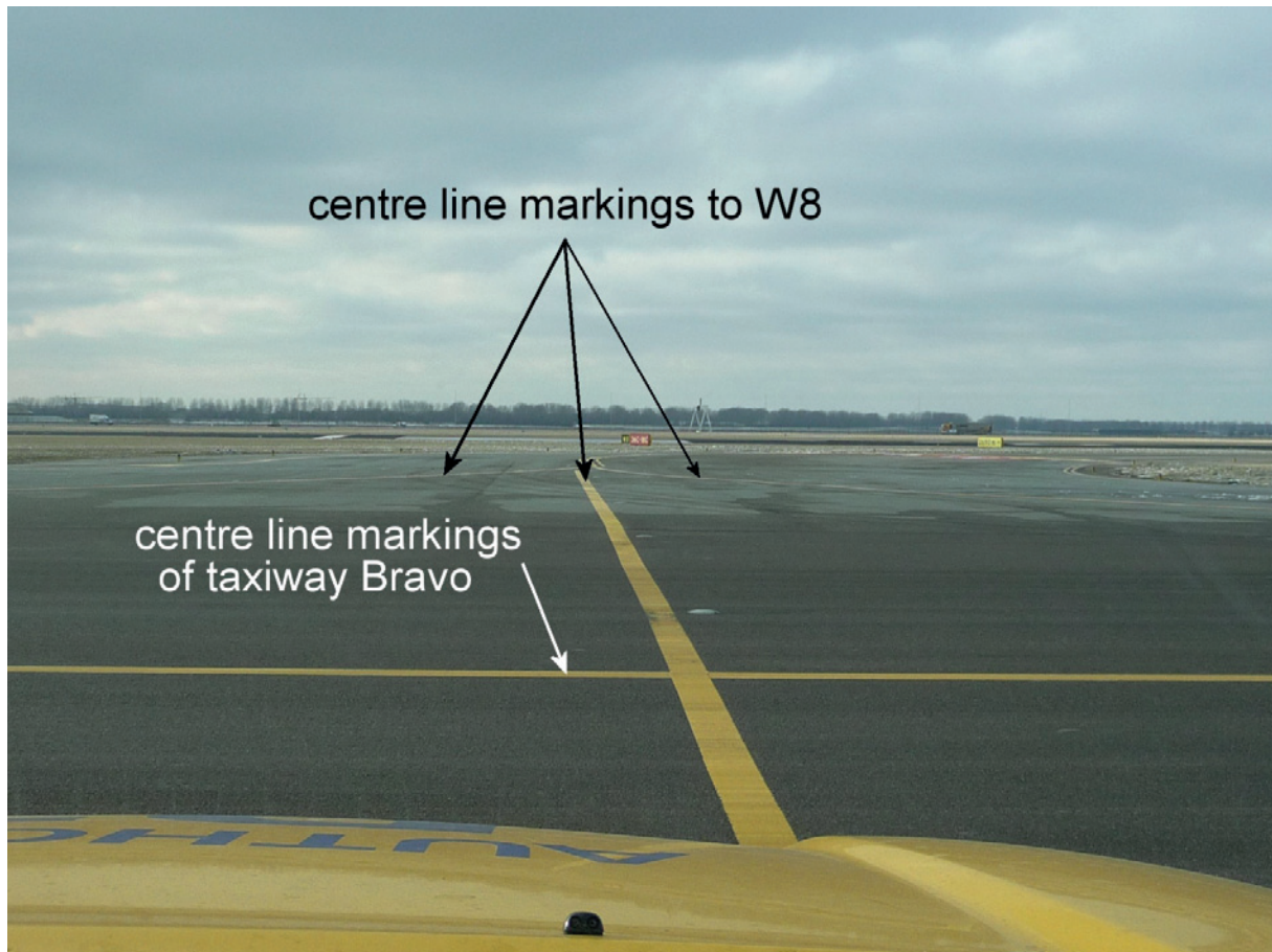
Figure 7: Yellow marking lines (centreline markings) during daylight on the intersection of interconnecting taxiway A25 with taxiway Bravo viewed into the direction of runway 36C.
