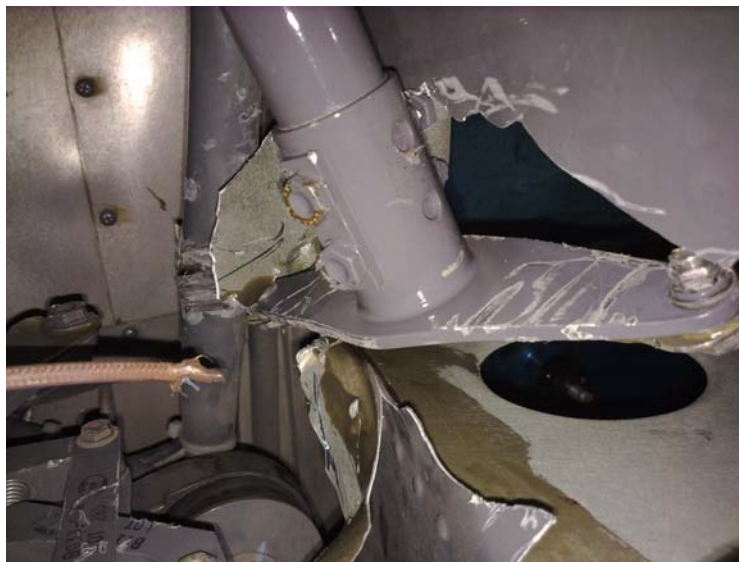
Figure 4: View of a destroyed forward yoke in main tank
