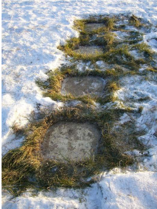
Fig. 5 Day marking threshold runway 04.
