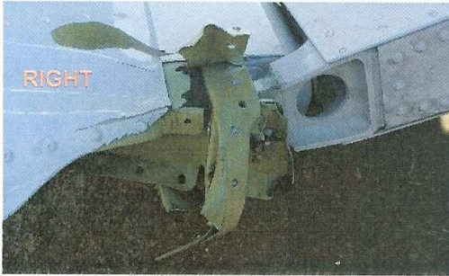
Photo 5: Right hand elevator damaged outboard hinge (digital)
