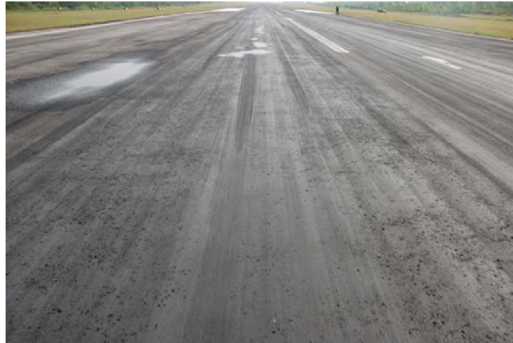
Figure 3: Rubber deposit on the touchdown zone runway 18.
