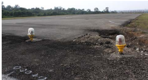
Figure 9: Final aircraft position after the aircraft has been removed
