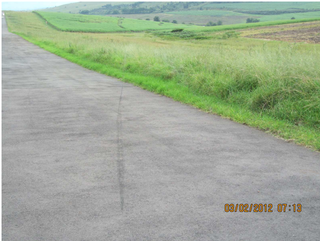
Figure 5. The left main tyre print on the runway surface.
