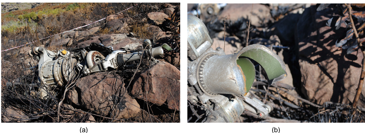
Figure 12. A view of the main rotor gearbox assembly (a) and a closer view of the main rotor drive shaft failure (b).
