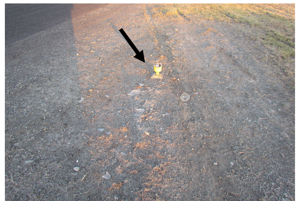
Figure 4 and 5, shows damage caused to the runway surface and light.
