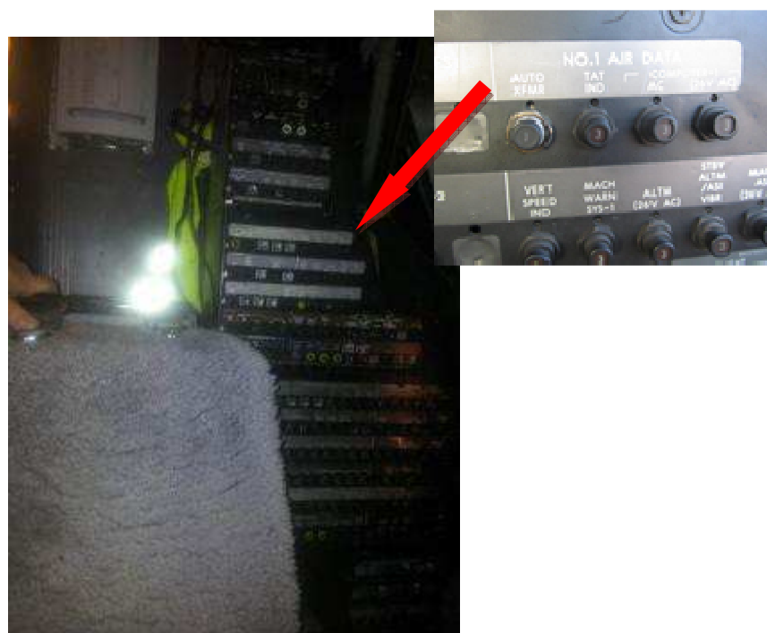
Figure 4: P28 circuit breaker panel showing #1 central air data computer system.
