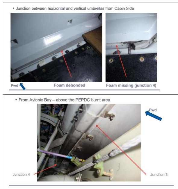
Figure 13. PEPDC protection- Foam condition and stains
