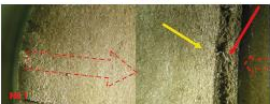
Photo 8: Fracture surface, No 1 bolt (stereo)
