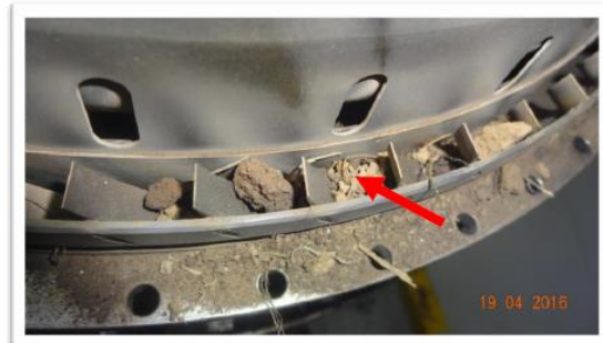
Image #20: Deposits of soil noted within the Deswirl Vane in the Combustion Section.
