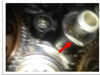
Image #6: Abnormal wear noted on the inside of the Accessory Housing in numerous areas.
