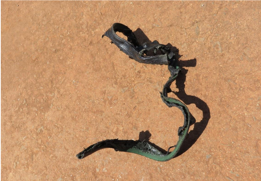
Figure 5. The air-conditioning drive belt that was found melted on the transmission platform
