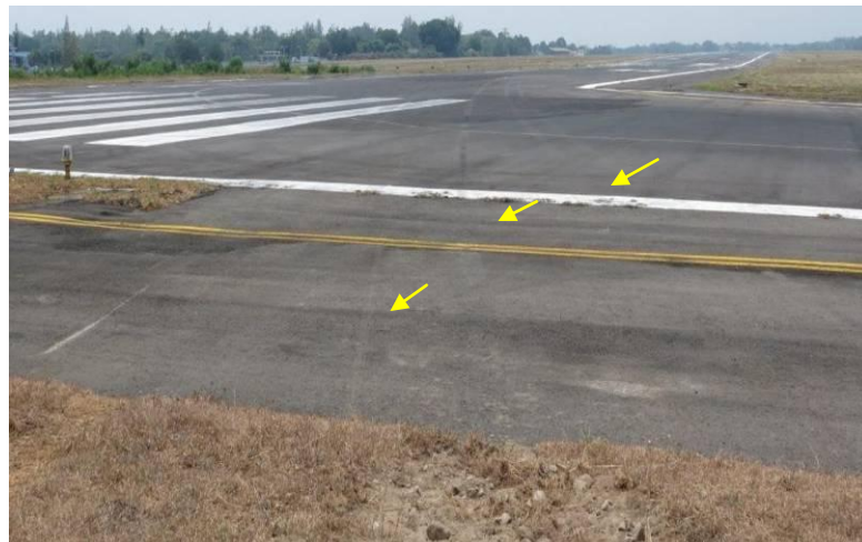
Figure 11: The main and nose wheel marks (indicated by arrows)
