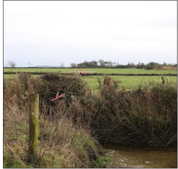
Photo No. 2: Close up of ditch with debris
