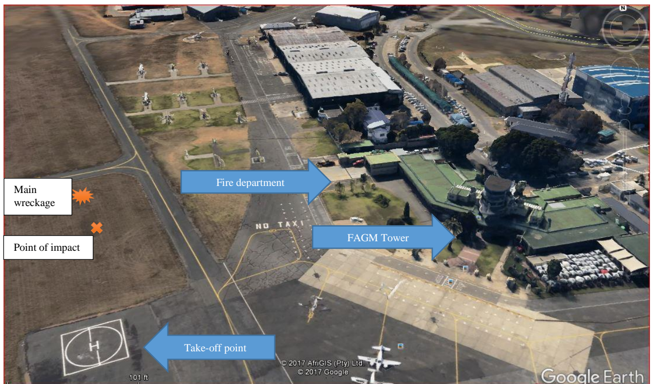
Figure 1: Google map showing position of accident site in relation to the tower.
