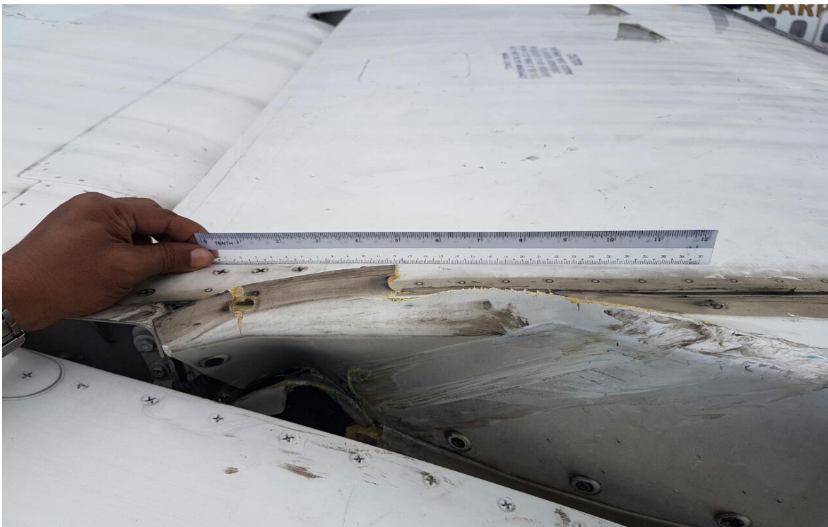
Figure: 7 The damaged upper skin of the RH Wing of ATR – 72-212A (600 version) aircraft
