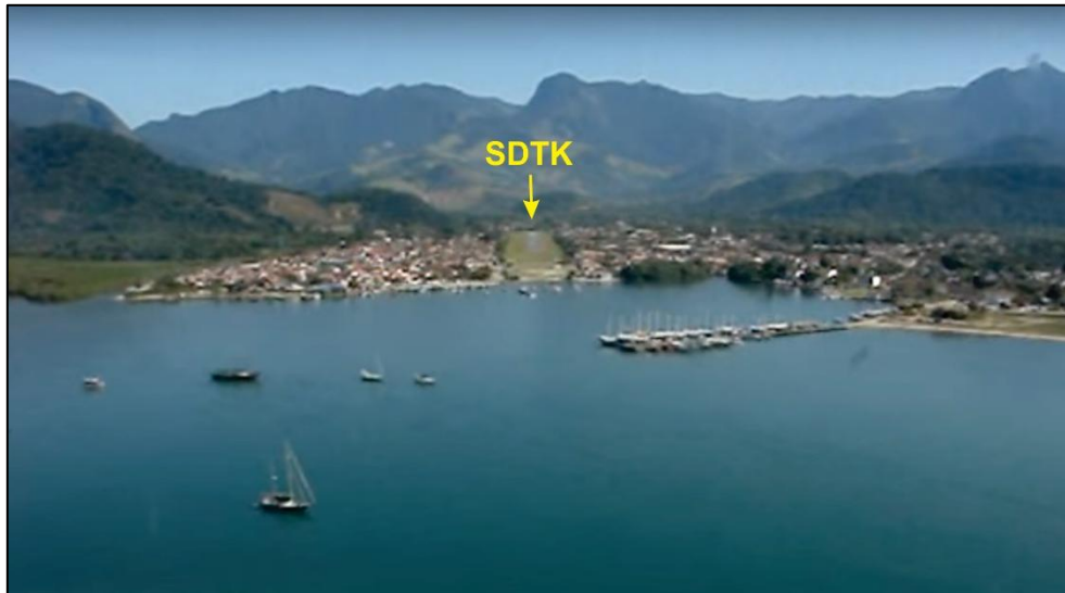
Figure 21 - View from the final to the SDTK threshold 28.
