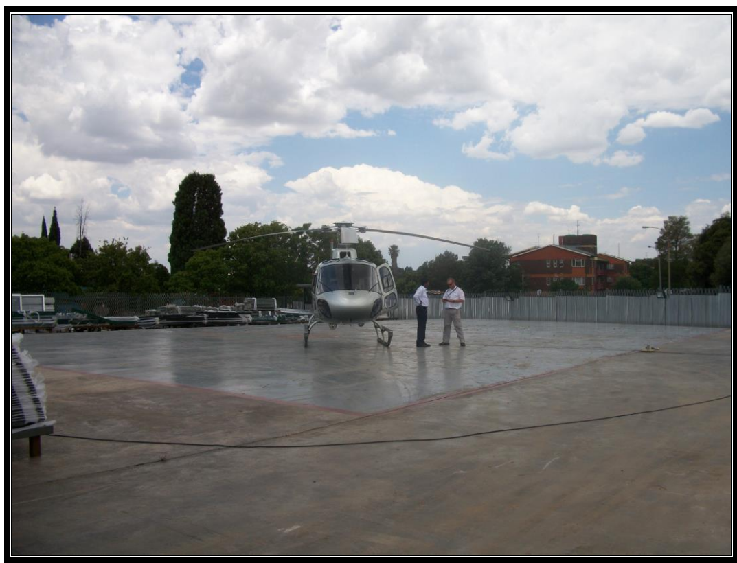
Figure 5: A photograph of the Spartan helistop with an AS350B2 parked on it.
