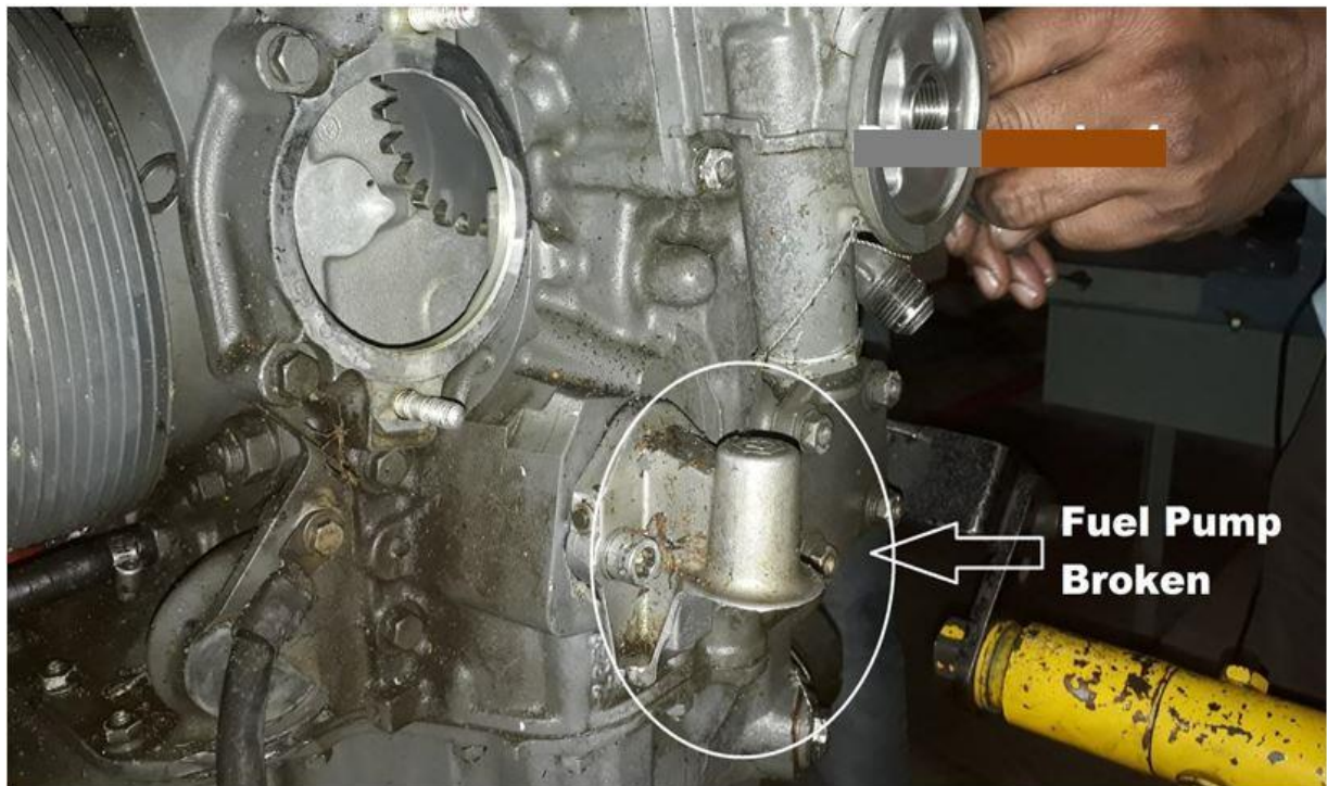
Fig: 29: Broken fuel pump
