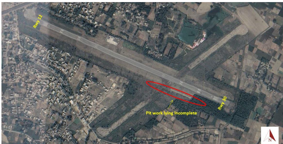
Fig 7: Layout of Faizabad Airport with incomplete mud pit highlighted
