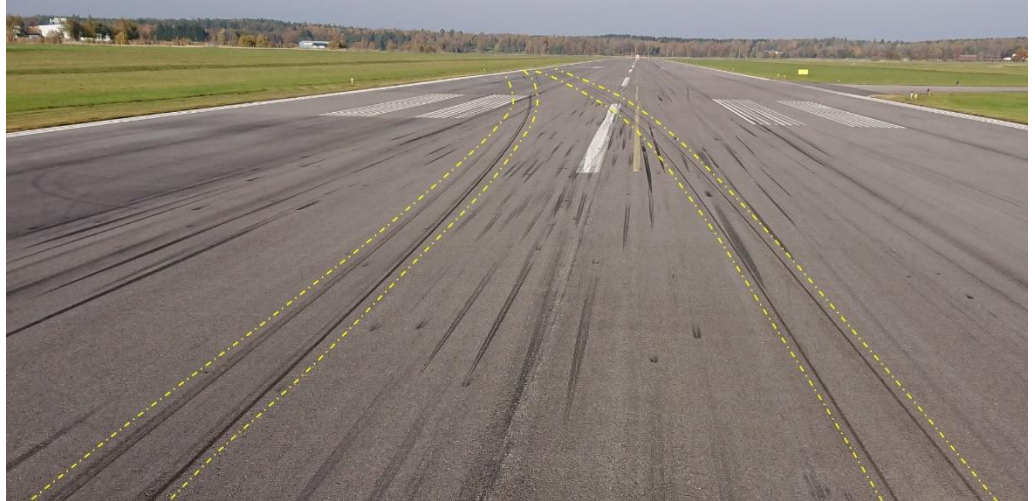
Figure 1. Tyre tracks in the landing direction towards the left edge of the runway. Photo: Trollhättan/Vänersborg airport.
