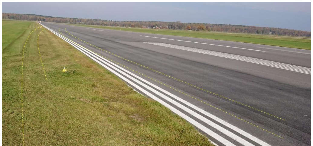
Figure 2. Tyre tracks going past the hit runway edge light and back onto the runway. Photo: Trollhättan/Vänersborg airport.
