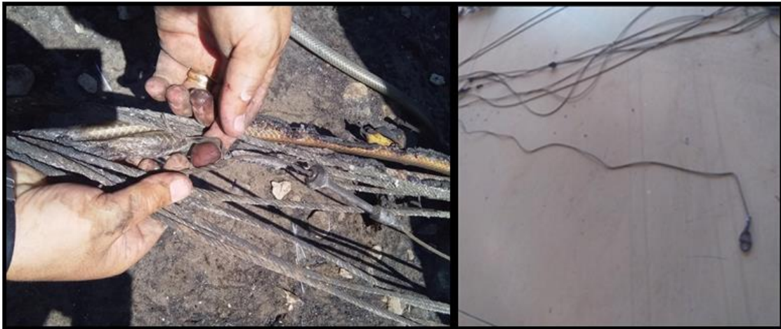
Figures 20: Damaged water-release cable and the Bambi Bucket holing cables.
