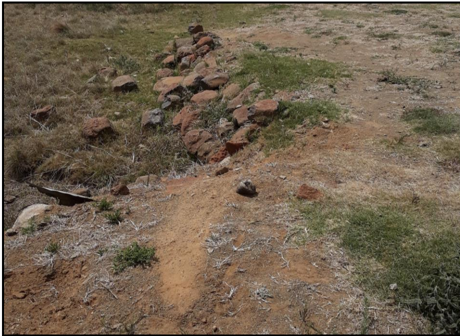
Figure 4: Rocky embankment and first point of impact.
