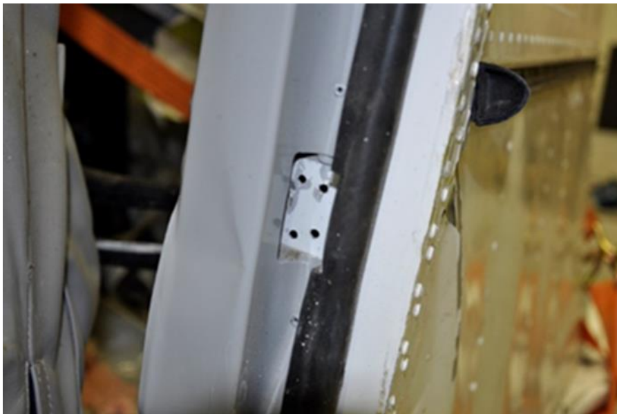
Figure 58. The picture shows that the pilot's door's locking catch was ripped out of its attachment.
