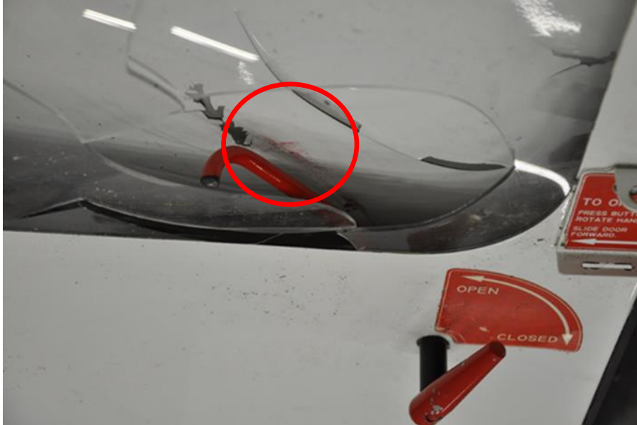
Figure 53. The picture shows an impact mark from the internal door handle on the outside of the fuselage.
