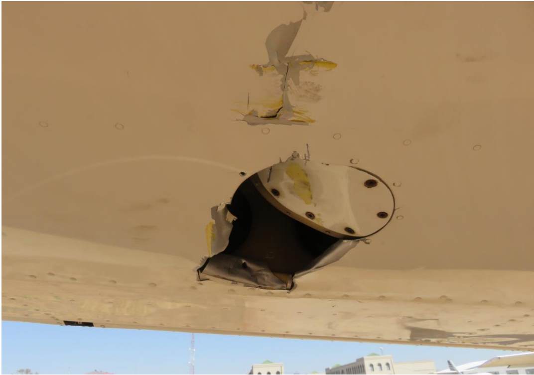
Figure 3: Damage caused to the right-wing lower skin following impact with a runway light.
