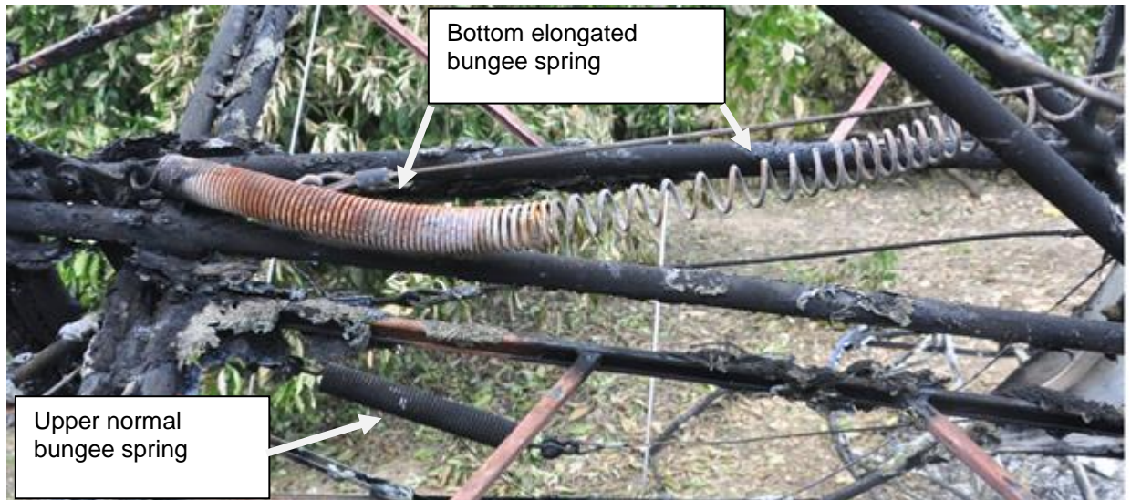
Figure 11: Elevator bungee spring cables.
