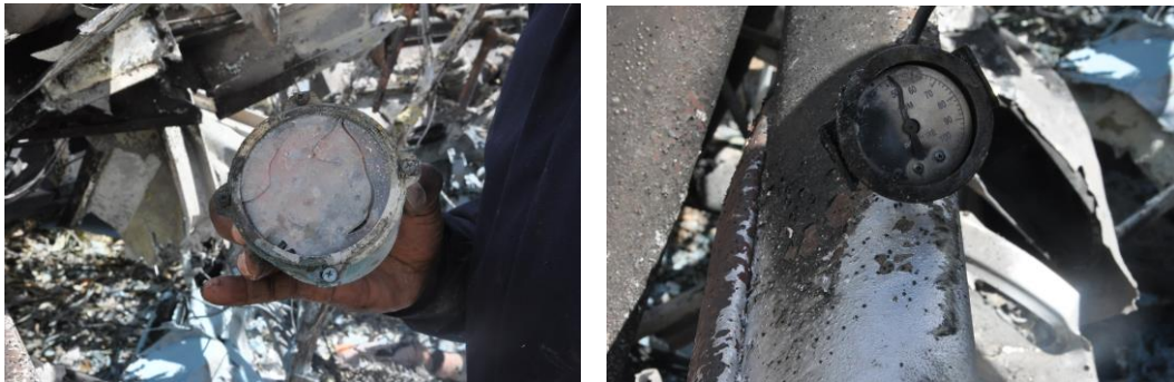
Figures 7 & 8: Damaged instruments.
