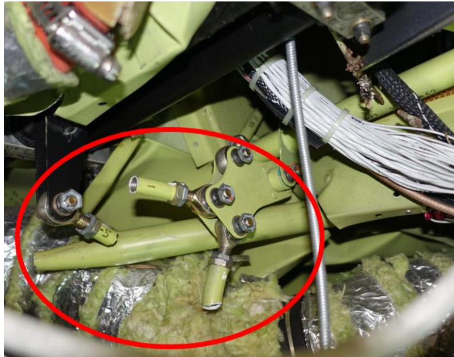
Figure 27. Broken push-pull tubes for the flight control system for yaw control in the area under the pedals.
