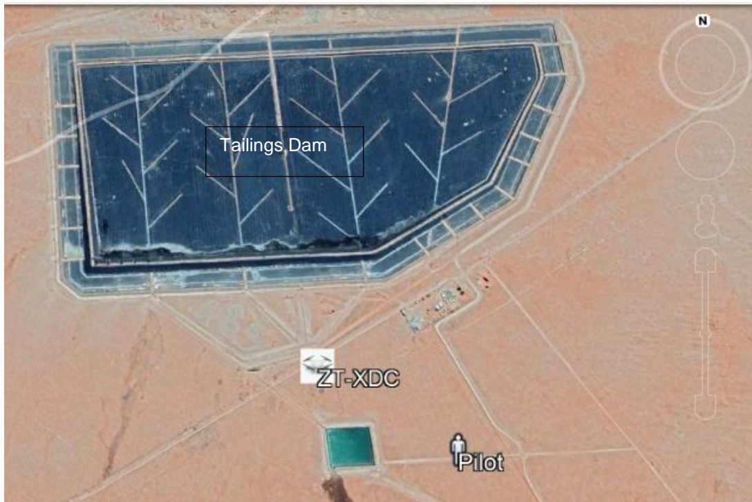
Figure 2: An aerial view of the accident site. (Source: Google Earth)
